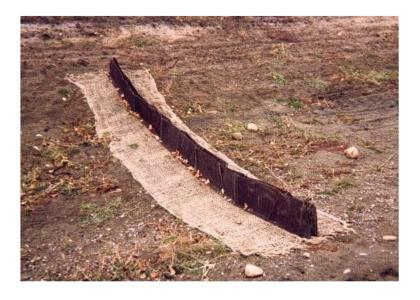
GeoJute Plus® installed as a strip channel liner under the EnviroBerm® Synthetic Permeable Ditch Barrier (SPDB)
